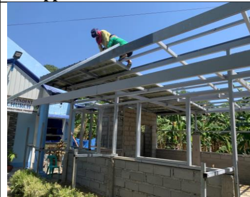
Philippines- main church addition
