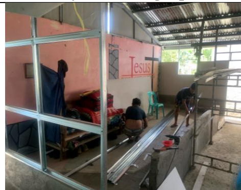
Building a room for Brother Zaldy, and storage space
